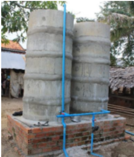
Picture 4. Drip Irrigation installation with elevated water containers
