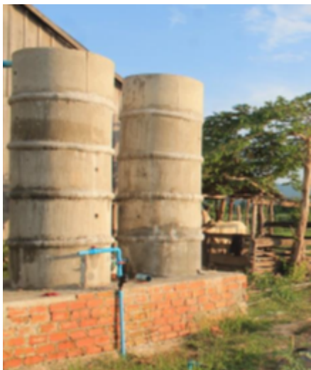
Picture 2. Modern water collection tanks, also called ring tanks.
